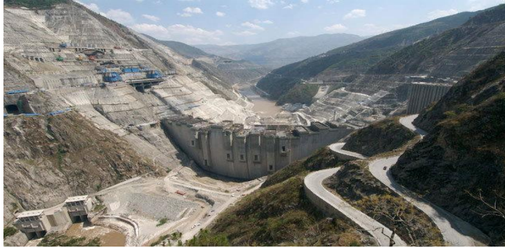
Xiaowan Dam (China) – 292 m tall – 4,200 MW installed capacity – 15 billion cumecs storage
